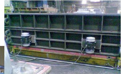
Compaction of concrete on a steel formwork using external vibrators from the NEG series
